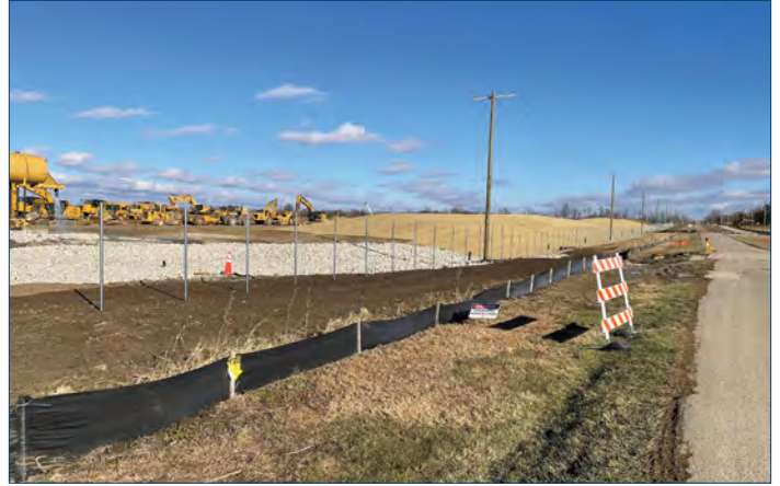
Perimeter fencing installation along County Road 375.
