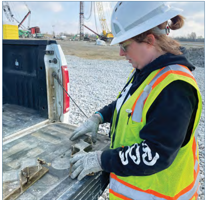
Katie Kessinger, testing technician, performs concrete quality checks on the LP1 site.
